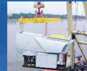
200 ton Lifting beam
