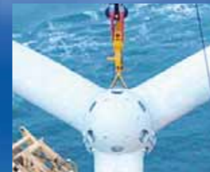
70 ton Rotor lifting equipment
